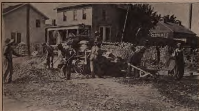
Street Paving, Delaware, Ohio. C. W. Riddle, Contractor
